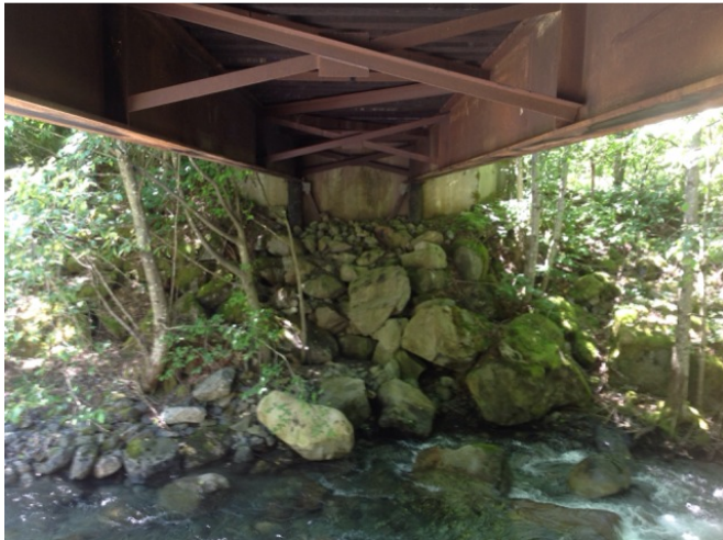
Left Bank Abutment when facing downstream
