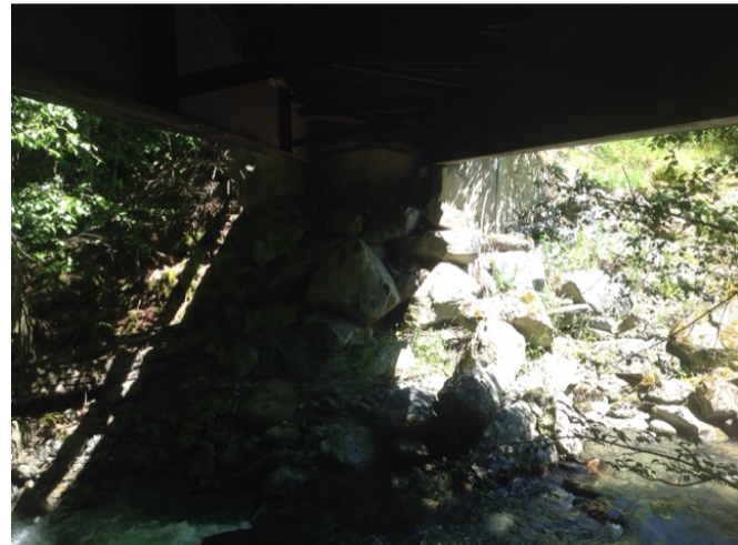
Right Bank Abutment when facing downstream
